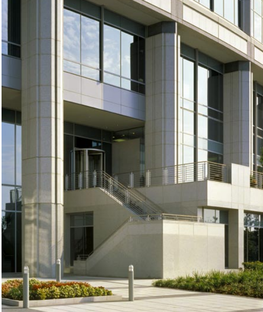
Architectural precast concrete spandrels and column covers were cast to match the Luna Pearl granite used on the lower levels of the Anadarko corporate headquarters. Photo: ©Richard Payne, FAIA Photographer
