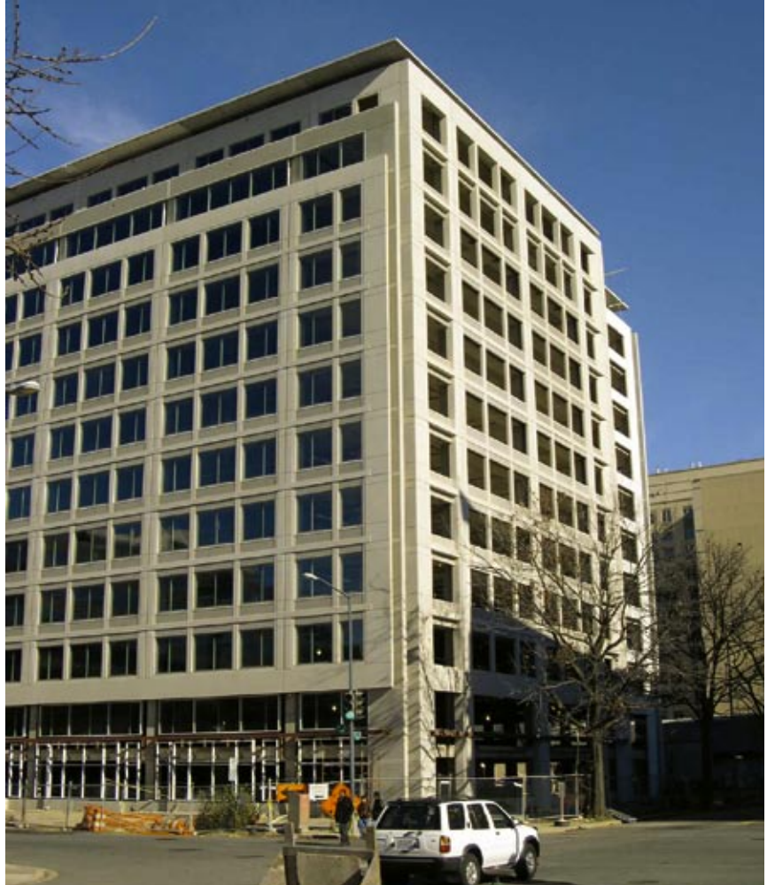
Patriot Square used two textures and colors of precast concrete panels to create a layered look for the speculative office building. The textures were emphasized by the inclusion of thin, jutting strips cast into the panels that run beneath the ribbon windows.
