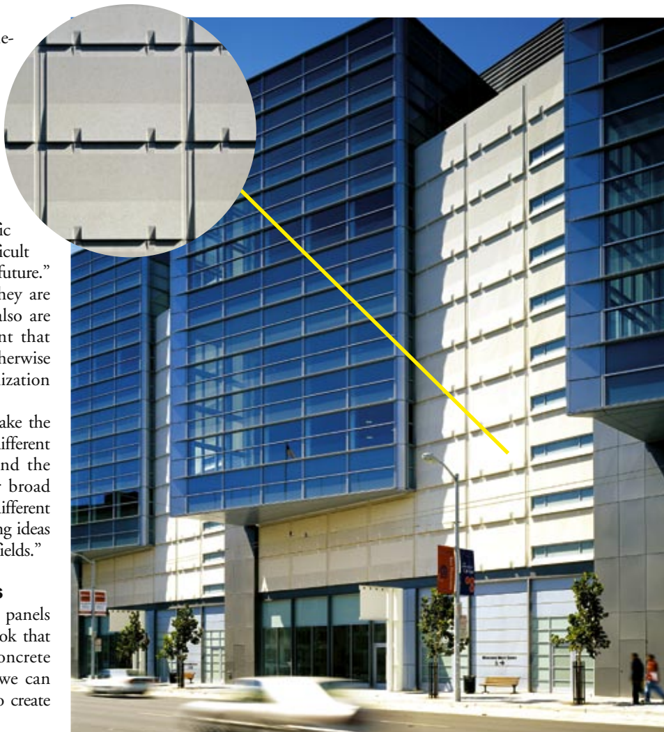
Architectural precast concrete panels and stair towers work in harmony with a large glass curtain wall and metal panels to give the Moscone West Convention Center a distinctive look that welcomes visitors rather than presenting the more typical closed-off face.
