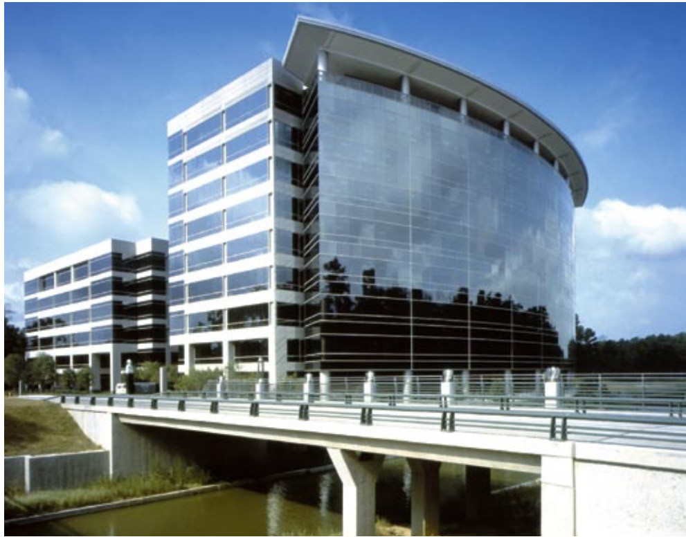
Waterway Plaza Two complements its companion office building, Waterway Plaza One, thanks in part to architectural precast concrete panels, which were used to clad the two buildings as well as an adjacent parking structure and freestanding stair and elevator tower. Photo: ©J. Aker; FAIA Photographer
